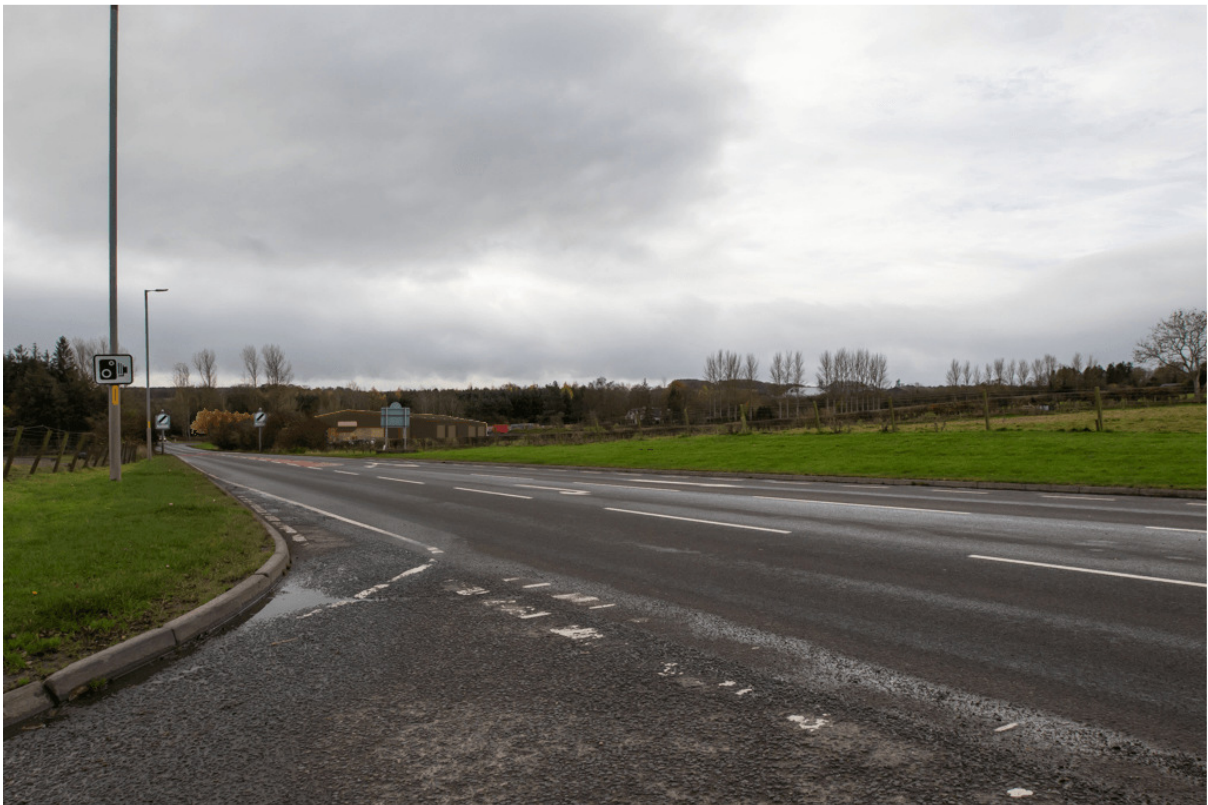
View from junction between A68 & A699
